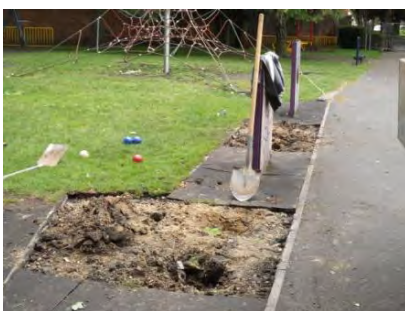
Old play panels dug out
